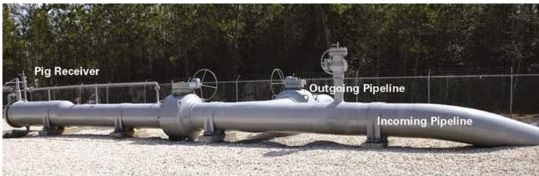
Example of a pig receiver on a natural gas transmission pipeline.
