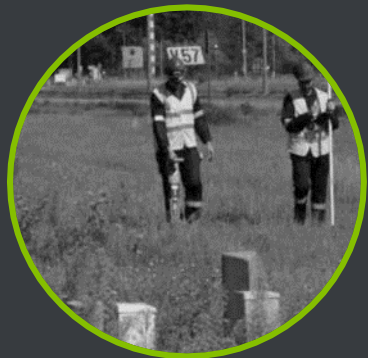
Pipeline Localization & Digitalization
