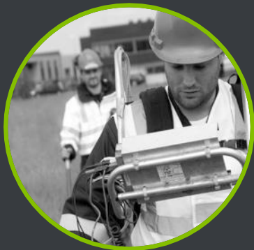
Corrosion Coating & Cathodic Protection Surveys
